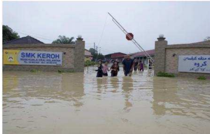
Fig. 7. SMK Keroh was flooded due to the overflow of Sungai Nal in Kampung Keroh in 2014 Source: BH Online (2014)
