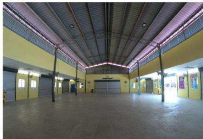
Fig. 8. Hall that used to accommodate flood victims.
