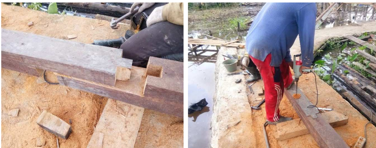
Fig. 6. The use of traditional wooden joint for new substitution element on the Hajjah Salmah house
