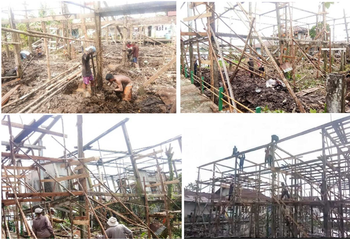
Fig. 5. Construction process on the reconstruction of Hajjah Salmah House. Re adjustment of house structure
