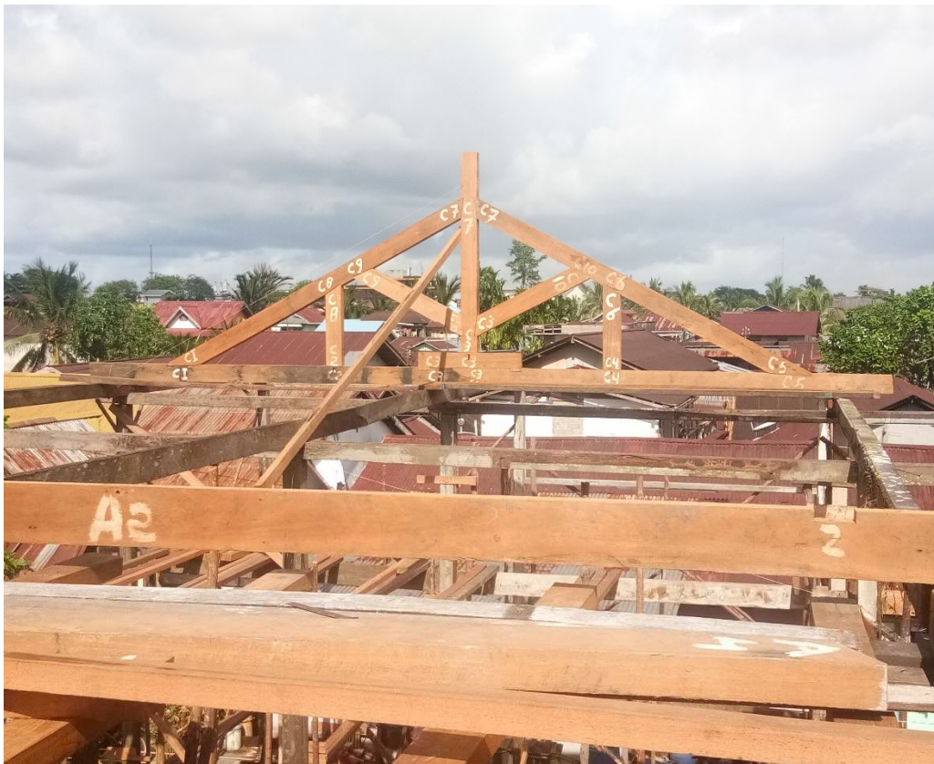
Fig. 7. Trestle structure for roof construction of the Hajjah Salmah house
