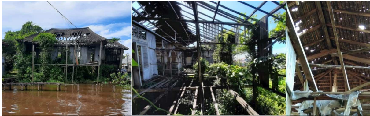
Fig. 2. Some pictures were taken in early 2019 about the house condition before reconstruction. The condition of structures was found to shift because of riverbank erosion and material decay.
