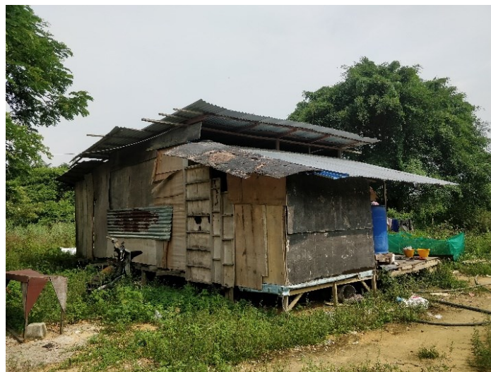
Fig. 4. Exterior View of the on-Site Temporary Workers' Accommodation With Poor Condition Source: Authors (2021)
