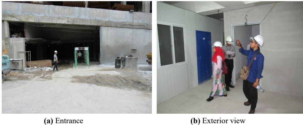
Fig. 3. The Entrance and Exterior View of the Bedroom for the Construction Workers Source: KLCH (2021)
